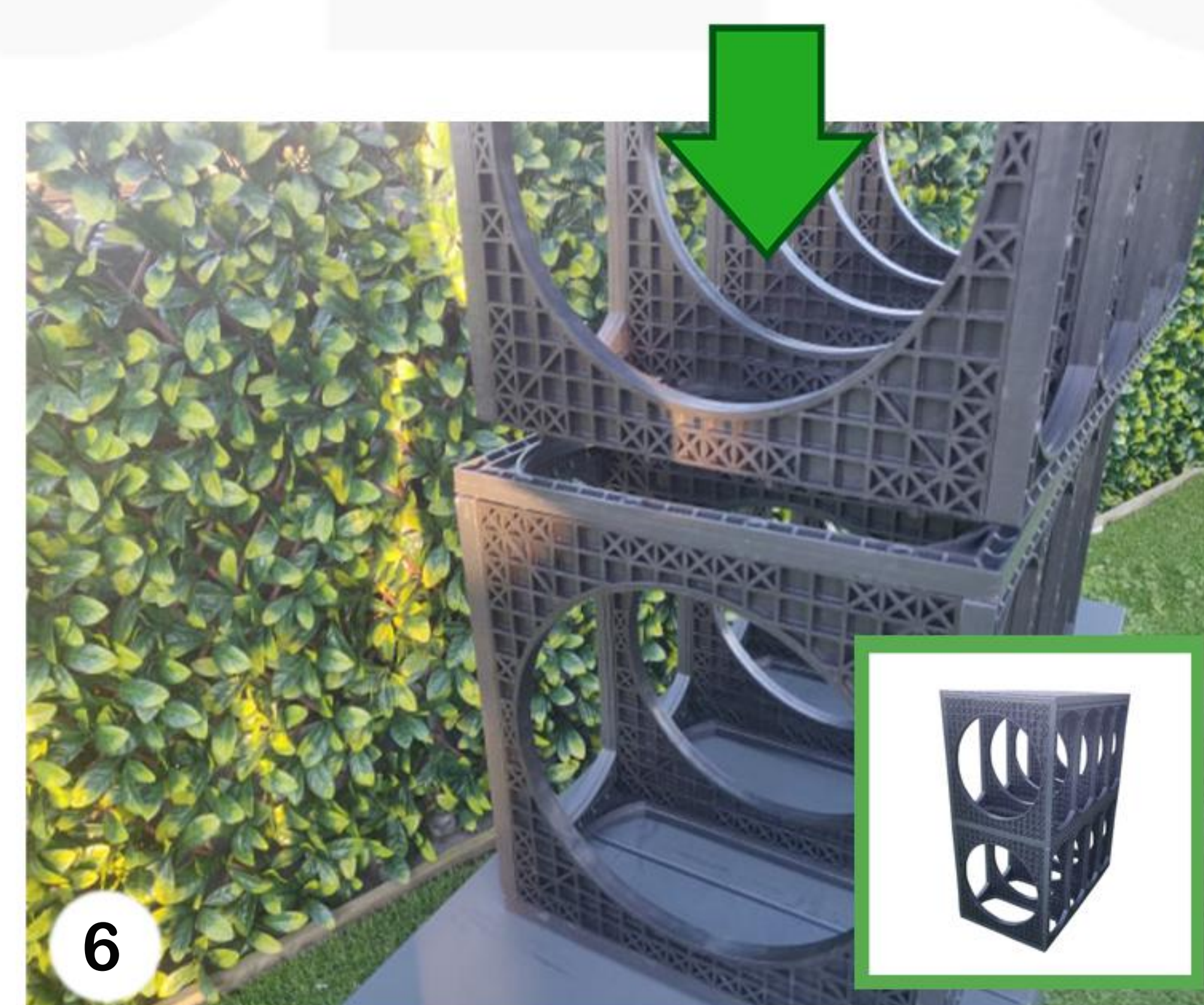
6 Place this crate on top of the shallow module you built (steps 1-4) open face down. You now have a double module – put this to one side.
