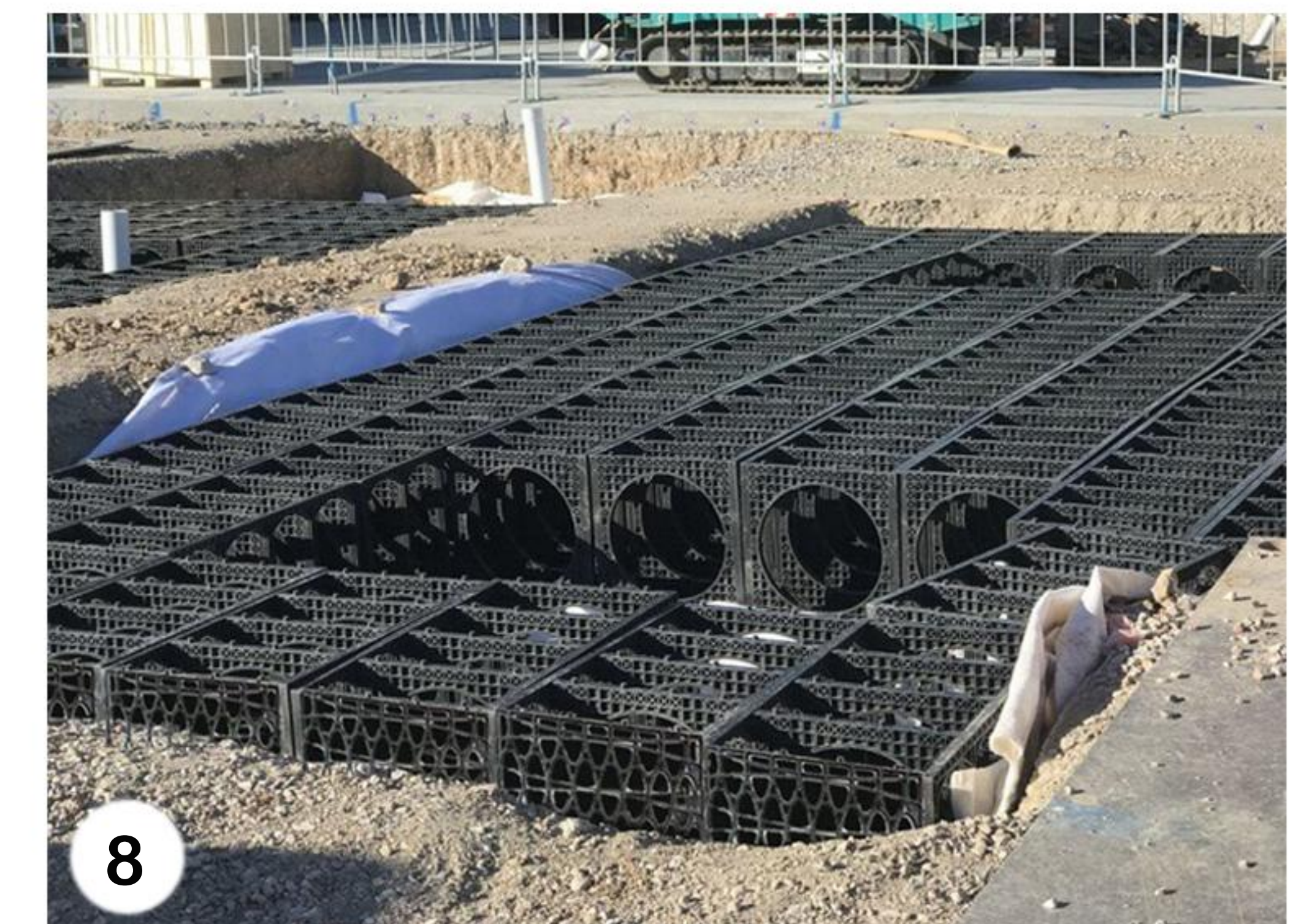
8 Add the crates to your excavation with the open tops. Fill modules with nutrient-rich soil. You can then attach the final Ellipse large closed plates on top of the modules.
